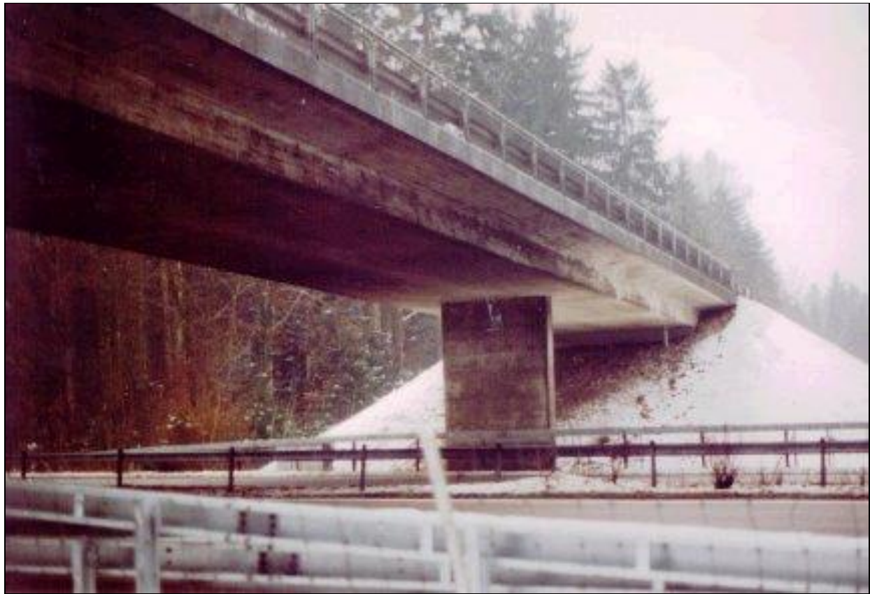
Z24 Bridge Viewed from the Bern-to-Zurich Highway A1
