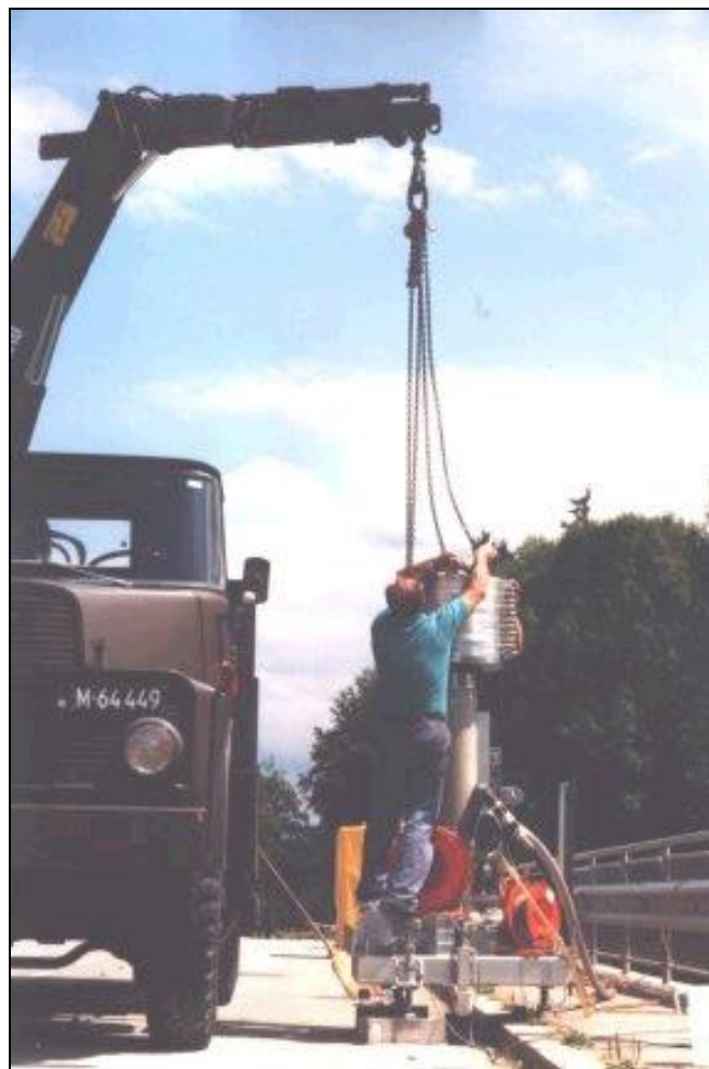
Installing one of the two shakers used to Excite the Bridge.
