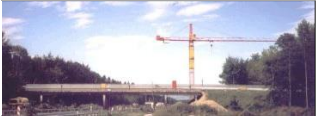
Z24 Bridge on the Bern-to-Zurich Swiss Highway A1.
