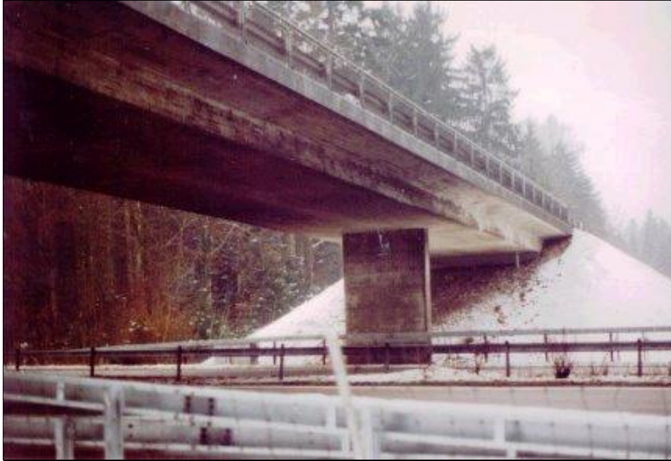
Z24 Bridge on the Bern-to-Zurich highway A1
