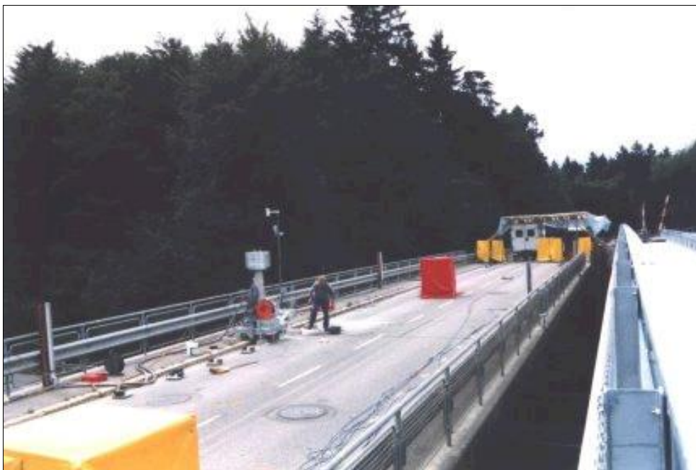
Deck of Z24 Bridge During Tests (The Replacement Bridge is Adjacent.)
