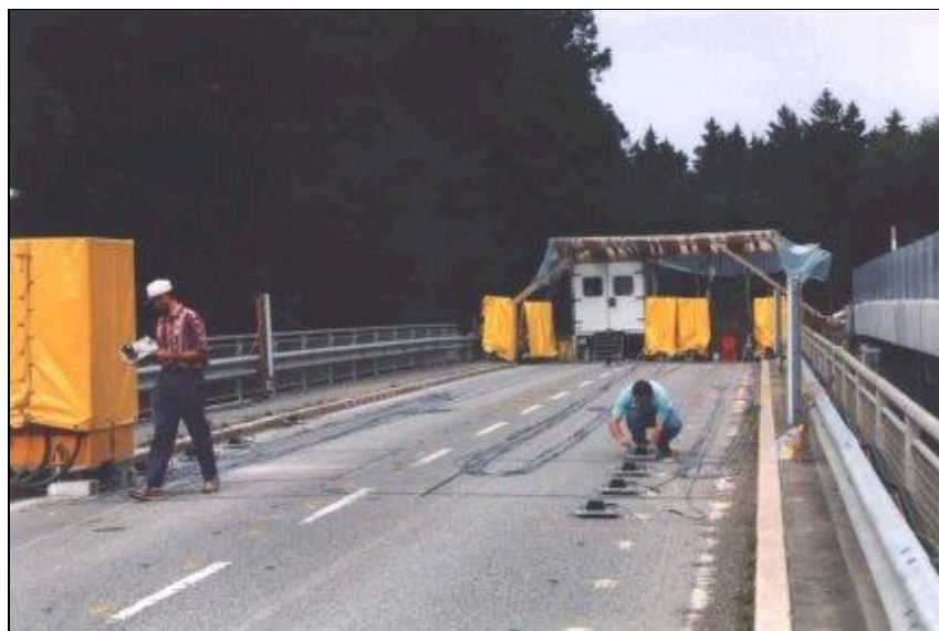
Installing the Accelerometers for one Measurement Set.
